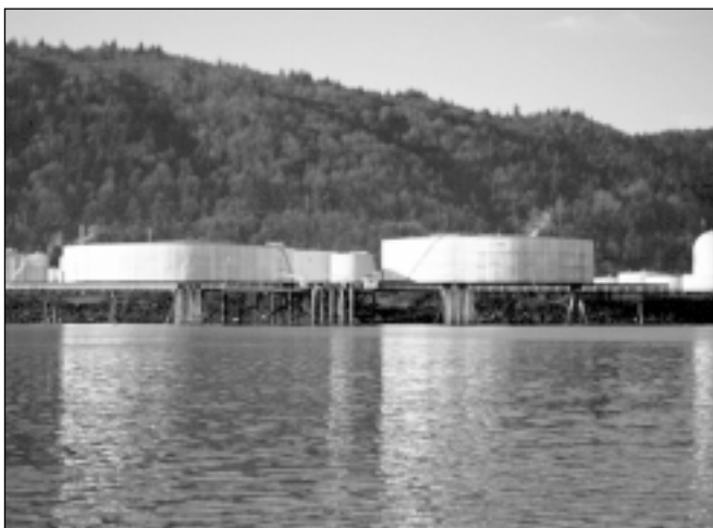
Industrial pollution continues to plague our river. The Portland Harbor is a federal Superfund site.
