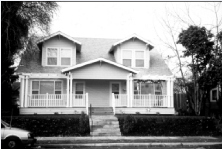
This duplex was designed to fit into a residential neighborhood. The density is twice that of a single-family dwelling, but it looks much the same.
