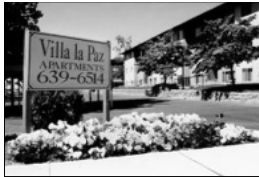
Villa la Paz, owned by Community Partners for Affordable housing, has 84 remodeled units and a new community center.
